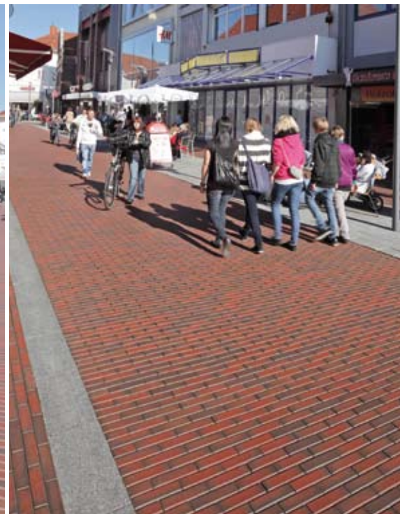
The Bockhorner Bunt pavers lend the pedestrian zone particular charm while, thanks to the hard-fired manufacturing technique, the surface is extremely robust.
