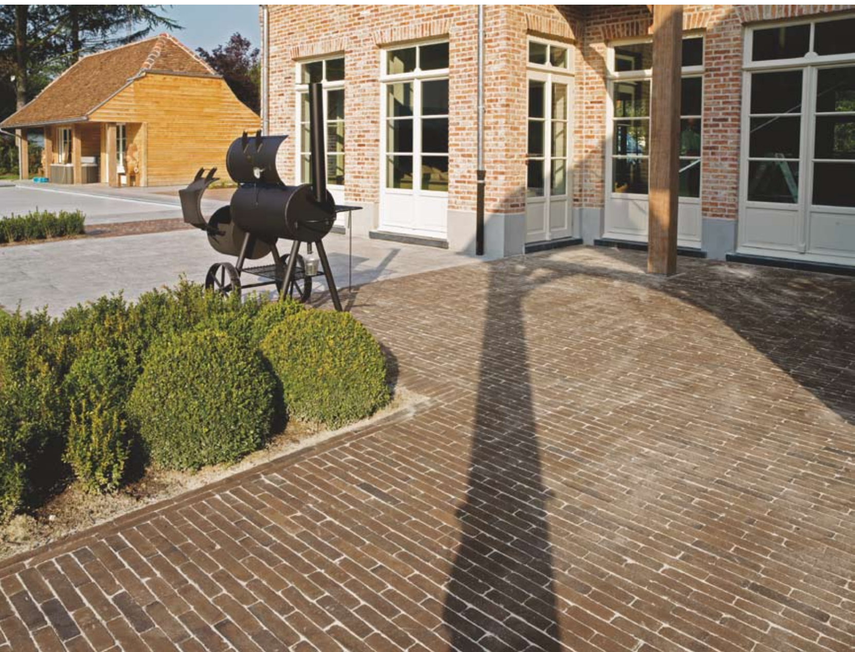
A double stretcher bond border serves as a transition to the gravel area or as edging for the lawn.
